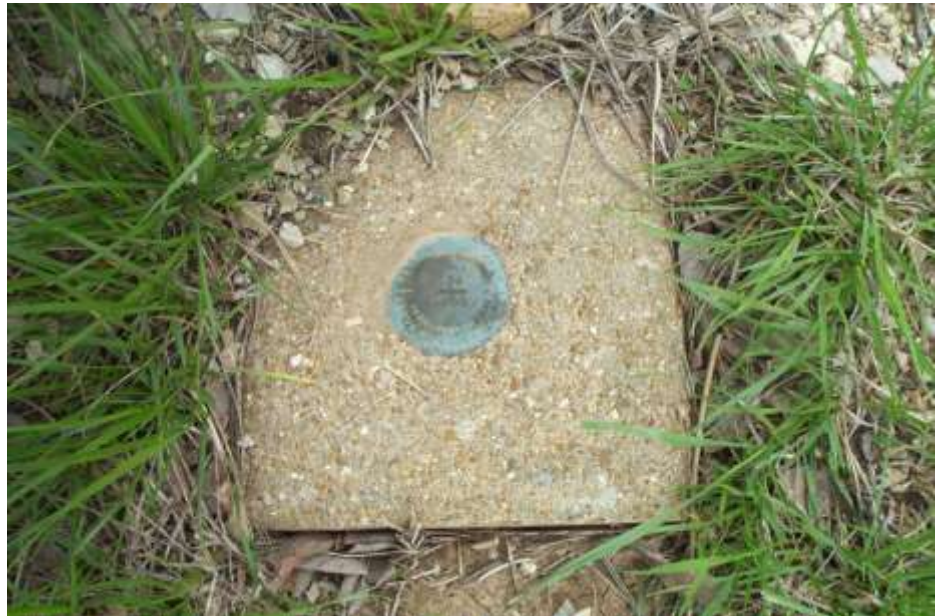
Poured in place concrete post
